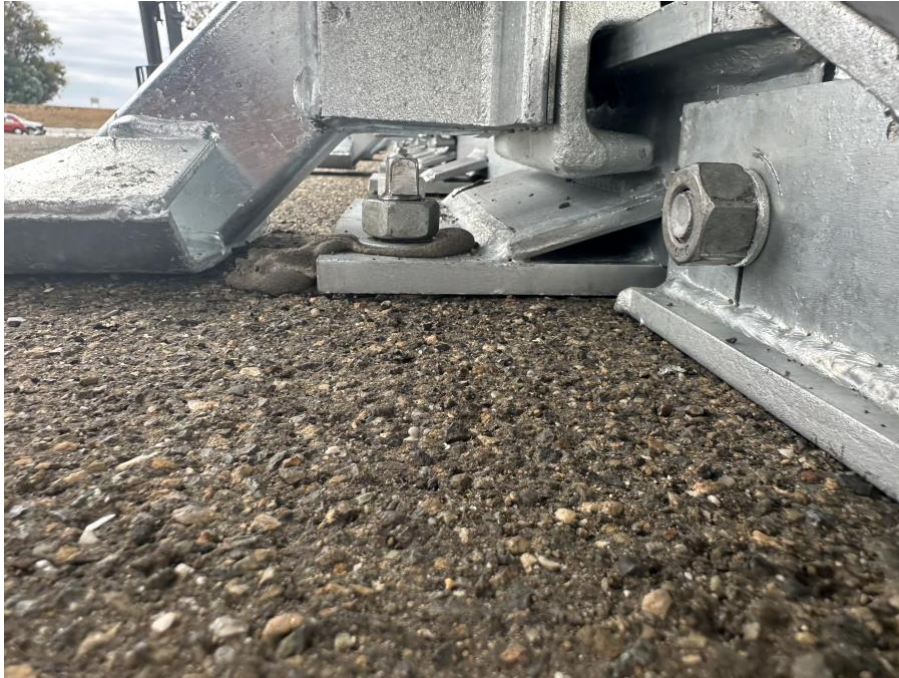
Image 5: Installed RoadLoc with QuadGuard Crash Cushion
