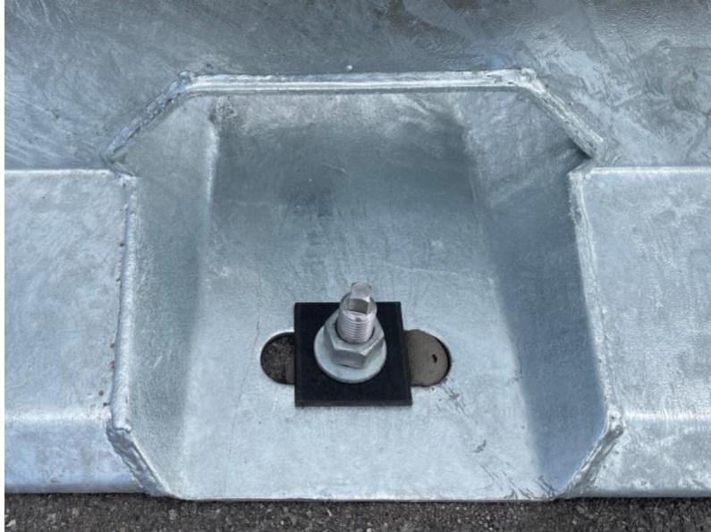
Image 4: Installed RoadLoc
